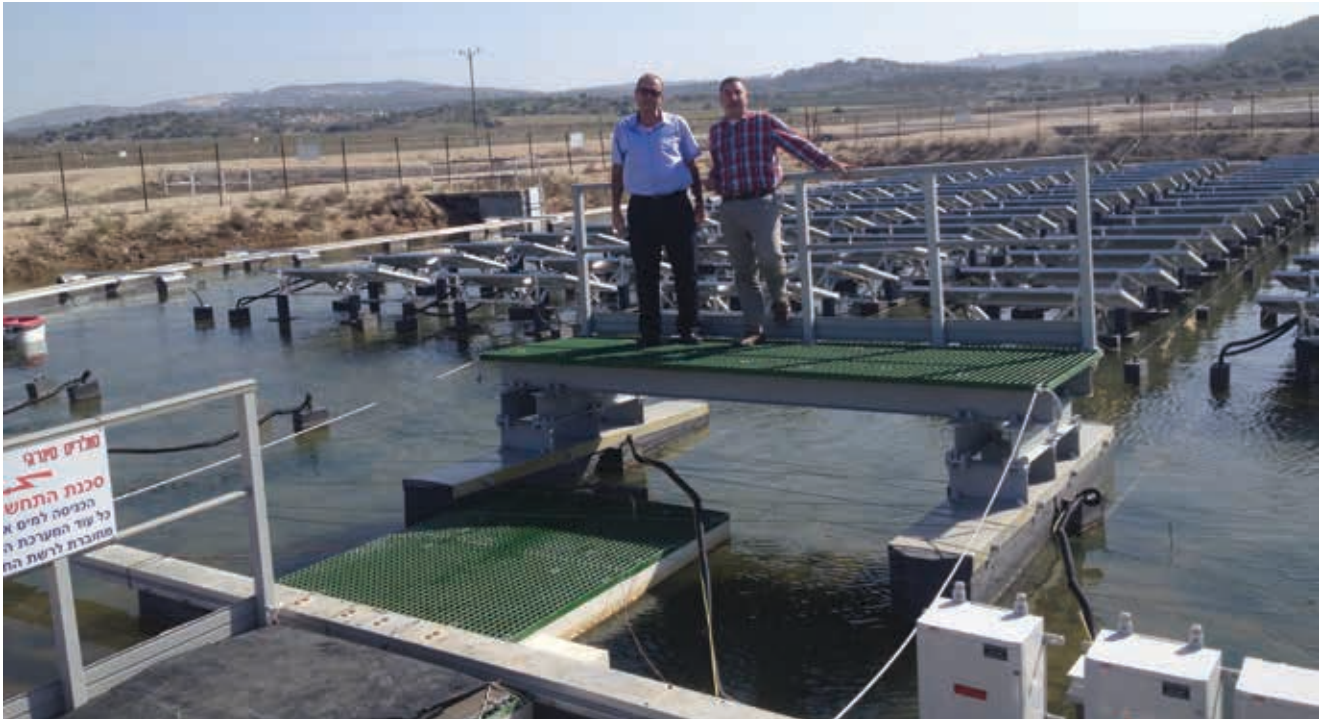
Floating Bridge: Floating Service Bridge for Module cleaning and maintenance
